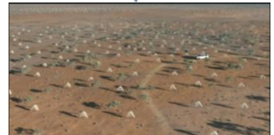
SKA2_LOW 250 x Low Frequency Aperture Array Stations
